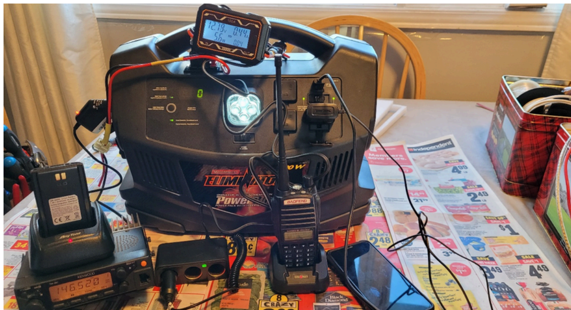
Photo 28 - Battery box final test powering multiple devices.
