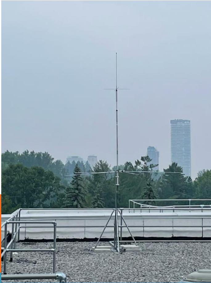
Diamond CP5H Trap Vertical Antenna 40M, 20M, 15M, 10M & 6M
