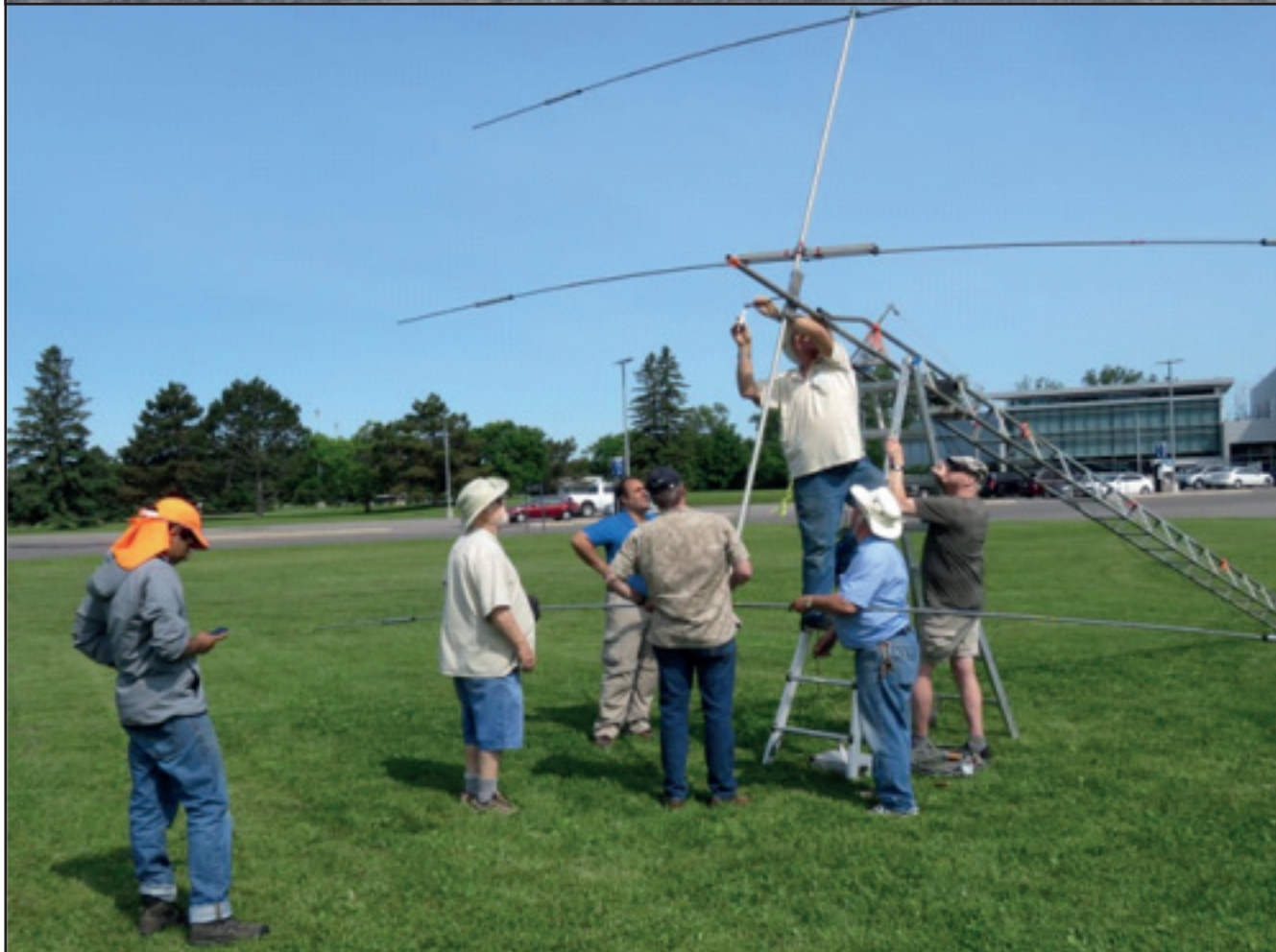
Getting ready to hoist the HF Tri-Bander
