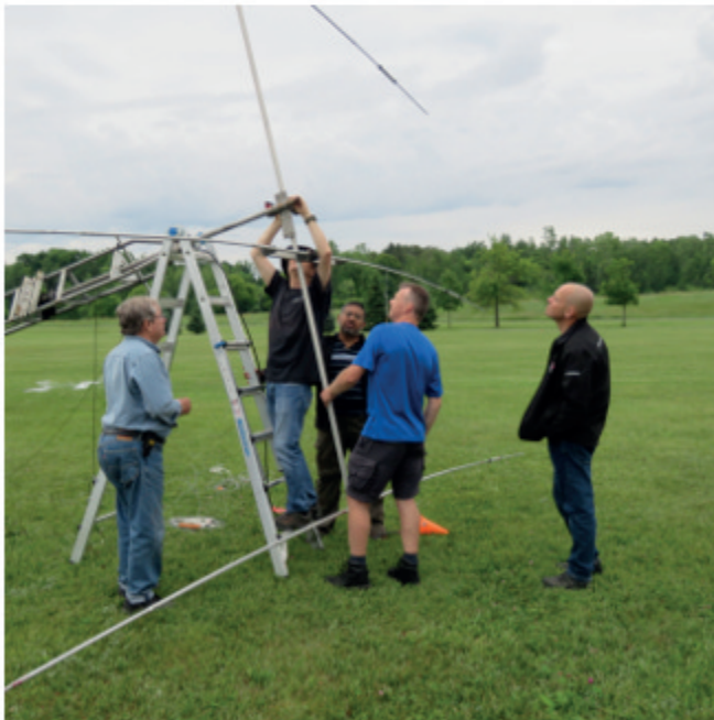
3 Band HF Beam ready to erect
