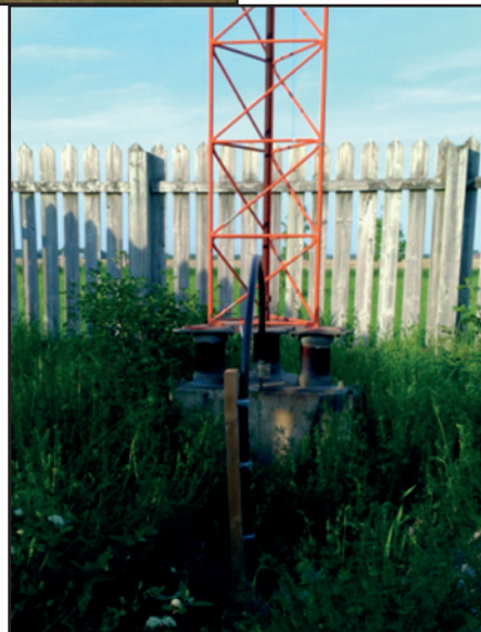
CHU's 3.33 MHz 1/4 wave vertical radiator (about 70 feet tall)
