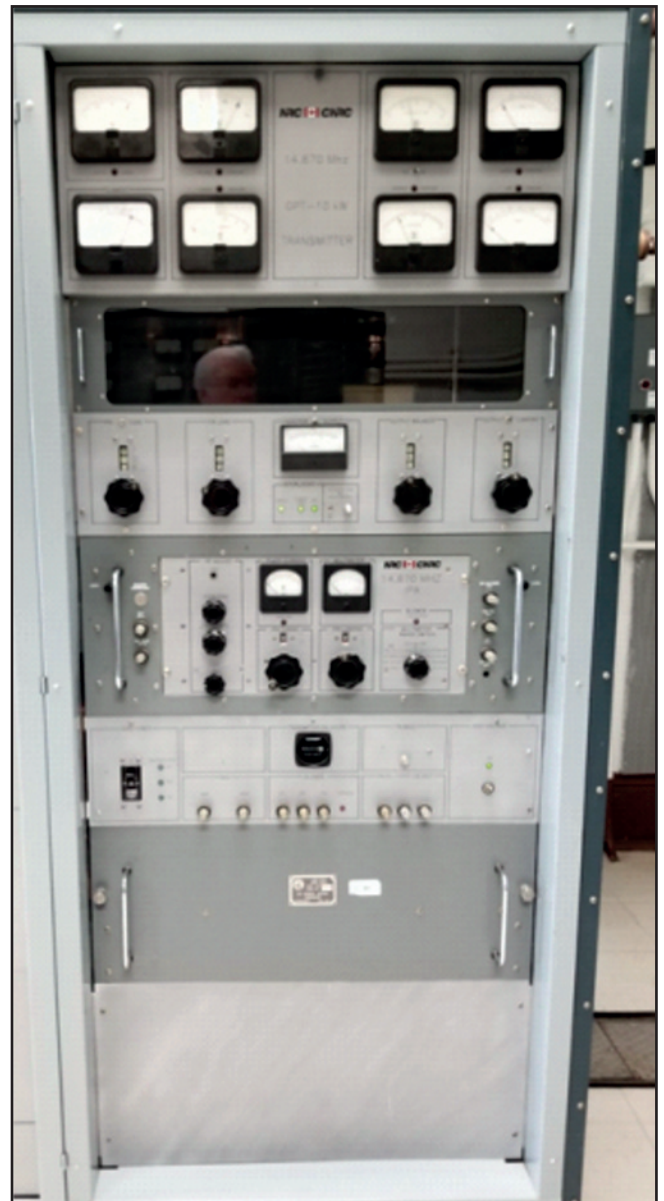
Active 10 KW transmitter operating on 14.670 MHz.
