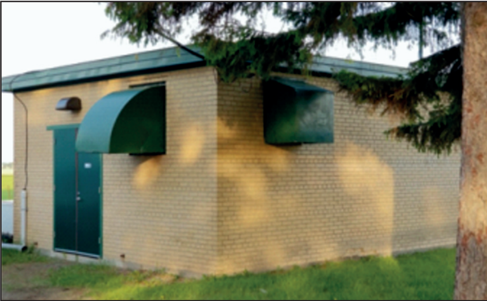
Standby Generator Building keeps CHU alive during power failures.
