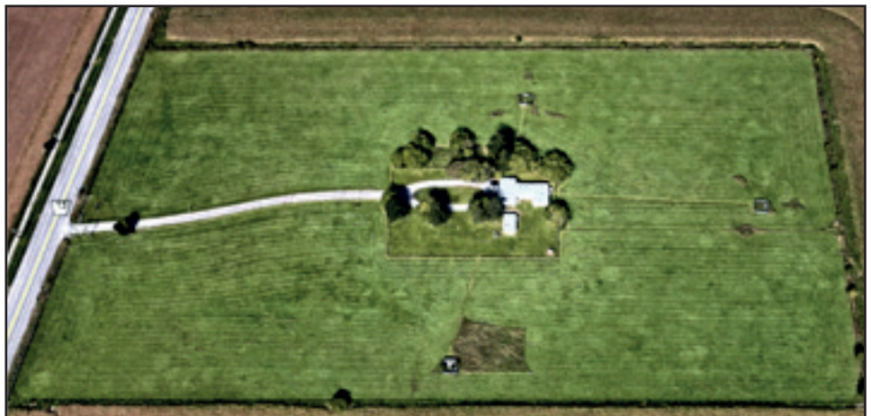
Aerial view of the CHU site courtesy of Google Earth. Note the location of the 3 antennas for the 3 bands of operation
