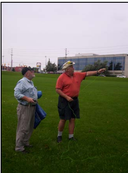
Figure 2 - Joe (VE3EUS) and Bob (VA3QV) installing a 80m dipole.
